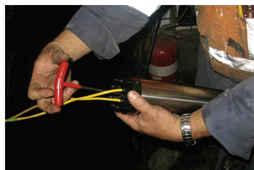
Connecting instruments to Top Logger in the field
